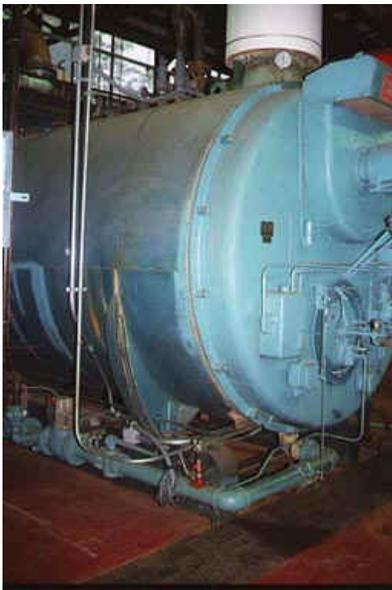
The most common water-level control and low-water fuel cutoff devices consist of two main components: a float chamber and an electrical switch operated by a float in the float chamber. A malfunction in either will prevent the cutoff device from operating. Malfunctions in the float chamber are generally the result of neglect; tampering and age most often cause failures in the switch and associated wiring.
